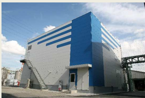
Modified Silica Gel manufacturing facilities (Amagasaki Plant)
