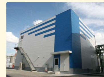
GMP-compliant modified silica gel production facility
