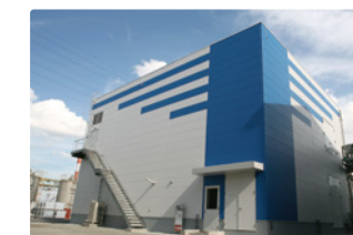
Amagasaki Plant Modified silica gel production facility
