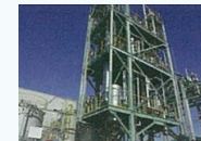
CABRUS™ production facility
