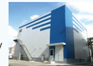
Silica gel production facility
