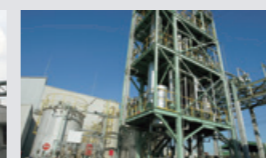
Production facility for modifying agents for low fuel consumption tires
