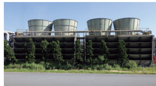
Cooling water recycling equipment (cooling tower)
