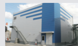
Silica gel production facility
