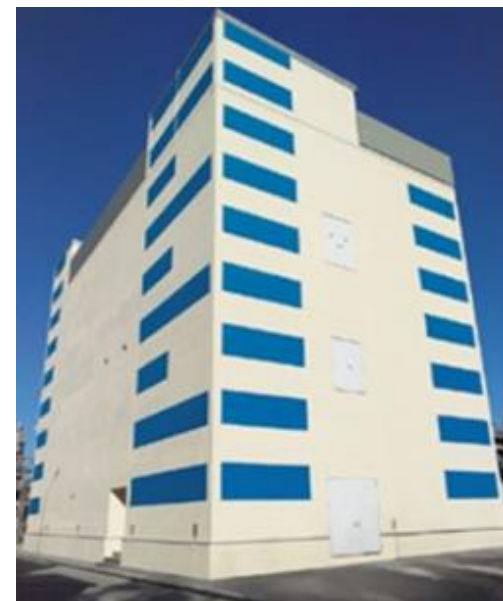
New facility “PI-3” at Matsuyama Plant (Construction completed in March 2023)
