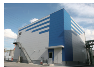
Silica Gel Manufacturing Facilities at Osaka Soda Amagasaki Plant
